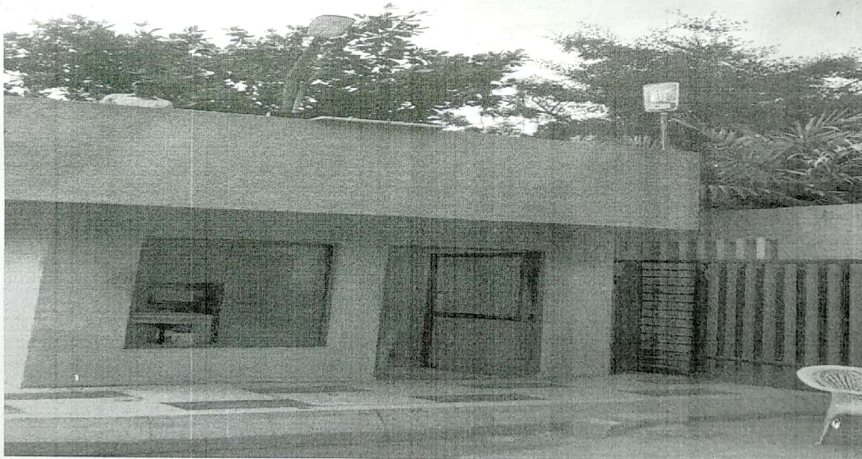
Solar Energy used for lighting at Security Room
