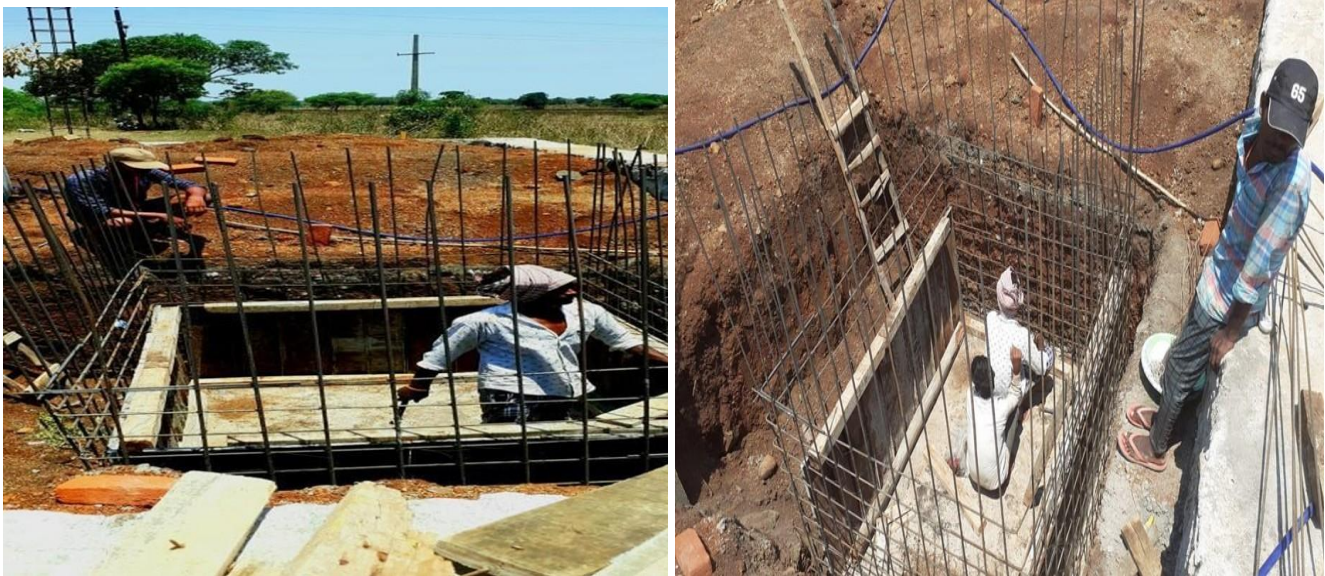
Students observed formwork construction of water tank
