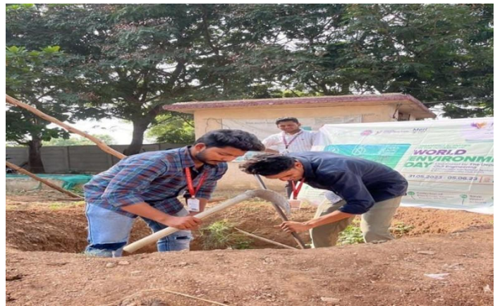
Students participating in excavation of compost pits
